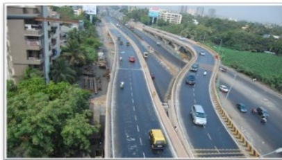
Amar Mahal Flyover
