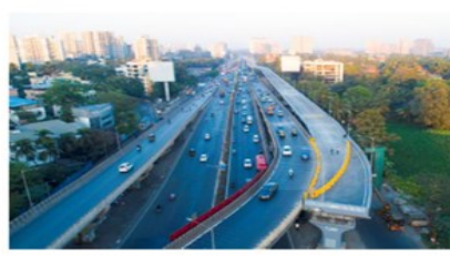
Chheda Nagar Flyover Part 1
