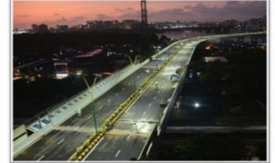
BKC - Chunabhatti Flyover
