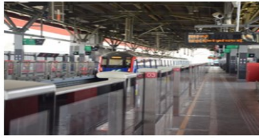
Mumbai Metro Line 7
