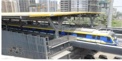
Mumbai Metro Line 2A
